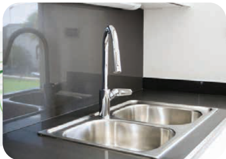
Steel Sink mounted on the black Granite Slab
