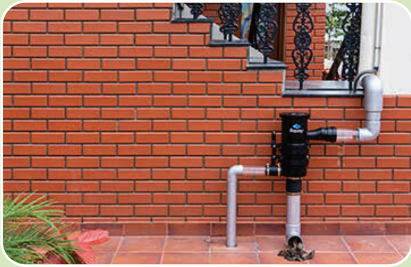
Rain Water Harvesting Filter
