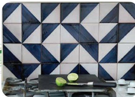
2ft Vetrified tiles provided over the working slab
